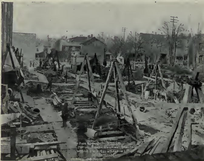
Fig. 1—Simpson Building, April 1.
